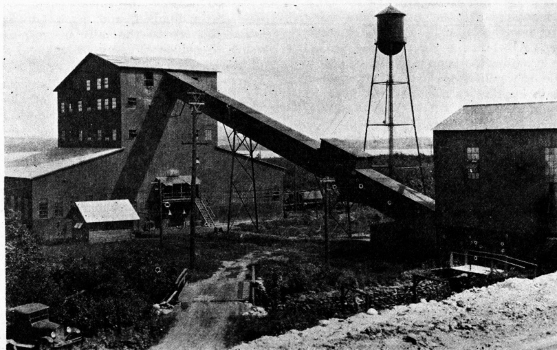
Hill-Trumbull Washing Plant, showing crusher house and conveyor bridge.
