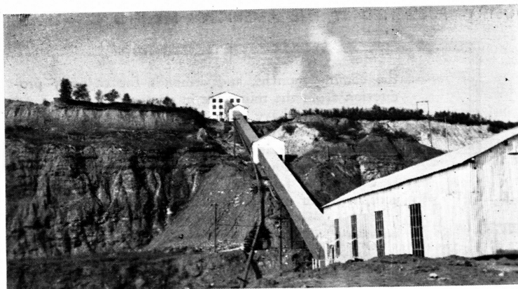
Canisteo Mine: Crushing plant in pit; belt conveyor gallery and transfer stations, leading to concentrator at ground level
